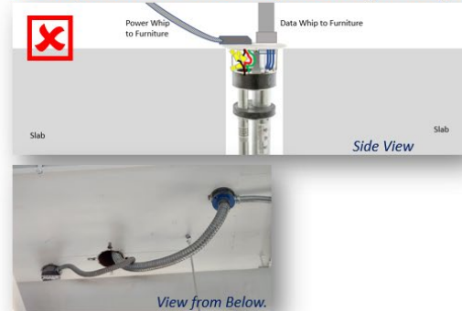
Example 2: Power and Data share one top plate that cannot be accessed once the data cables are pulled straight through.
