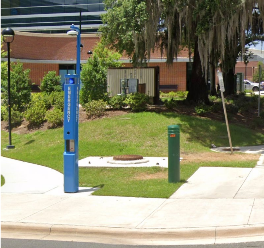
Figure 2. Bollard with cover next to blue light telephone.
