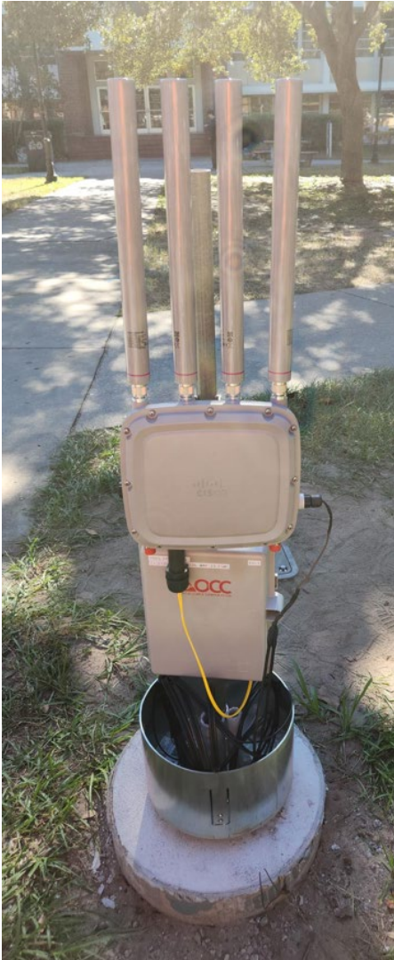
Figure 1. Bollard with Cisco wireless access point and fiber LIU.
