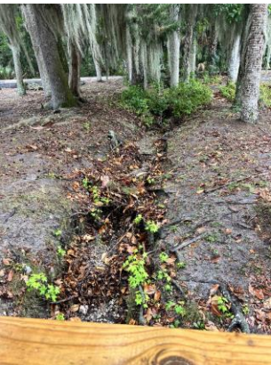
Swale at Bridge
