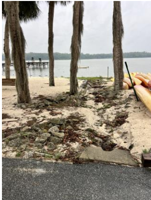
Swale at Lake
